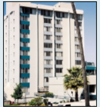
St. Paul's Manor follows the John A. McColl Family Health Center and the Community Care Center in undergoing a new paint job.
